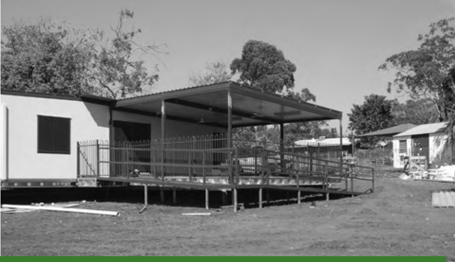
Milikapiti Creche being assembled at the site
