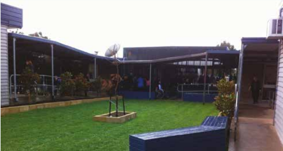
Melton Specialist School's upgraded facilities.
