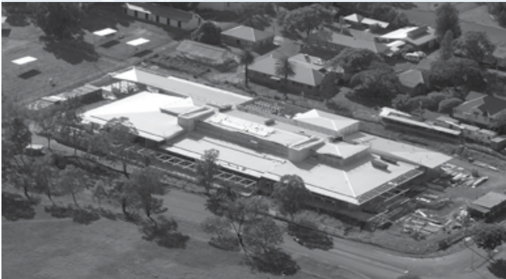
Construction of the Veterinary Hospital for the School of Veterinary Science.
